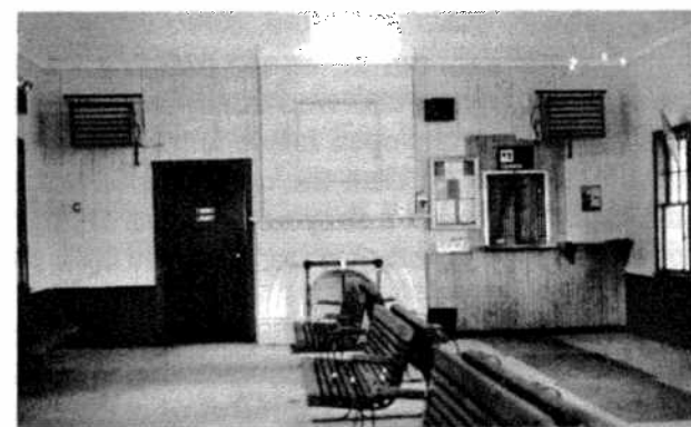
Views of the 111th Street Station (top to bottom): looking northwest across the tracks, the north baggage area, the main entrance portal, and the interior waiting room and its arched brick fireplace.
